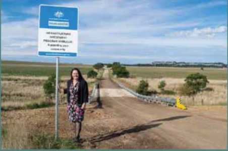
Rokewood Bridge upgrade ($541,000) Golden Plains Shire, Victoria.
